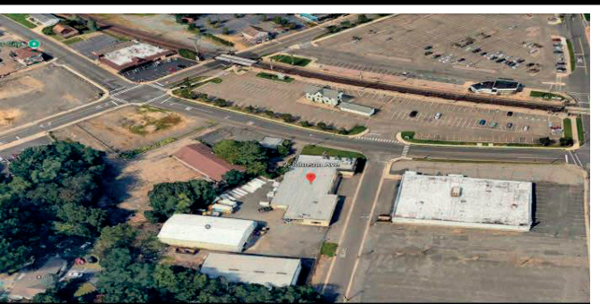
MATAWAN – FOR LEASE 8,500 +/- Square Feet – Warehouse/Showroom Two loading docks – Fenced Lot
